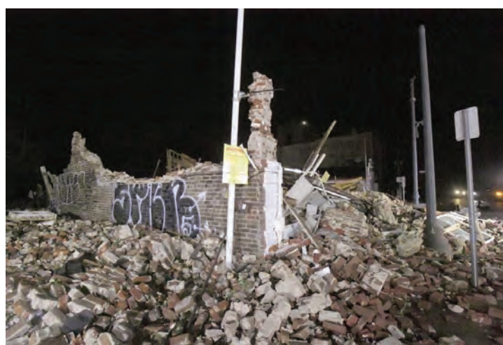
A collapsed historical building is seen on S. Rampart St. in New Orleans, La., early Monday, Aug. 30, 2021. Hurricane Ida became a tropical storm as its top winds slowed over Mississippi on Monday. (Max Becherer/The Advocate via AP)
